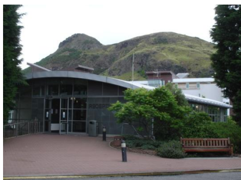
Figure 2: Conference Centre with Arthur's Seat in background
